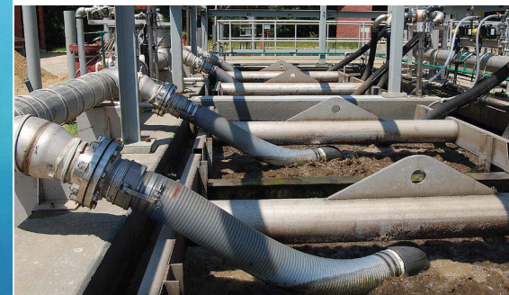
Aqua-Aerobic® MBR System at Riverhead, NY
