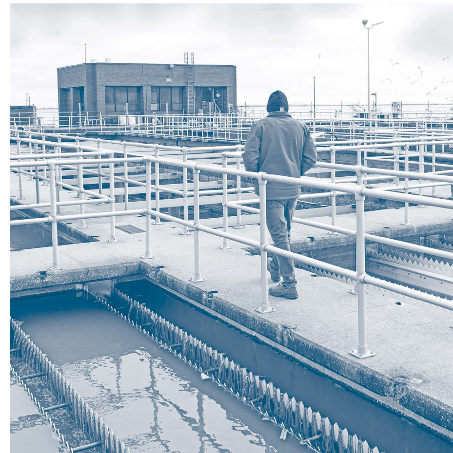
The Bergen Point Wastewater Treatment Plant uses an activated sludge process with 40 mgd design capacity and plans to expand to 50 mgd.
