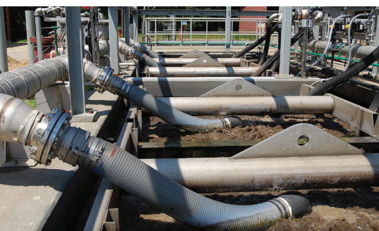
Aqua-Aerobic® MBR System at Riverhead, NY
