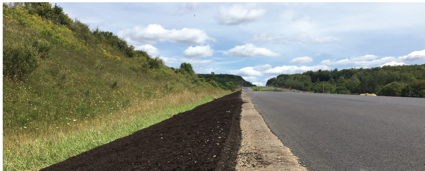
Biosolids compost being applied for miles along the side of a New York state highway project to promote the establishment of vegetation. Photo: Denali
