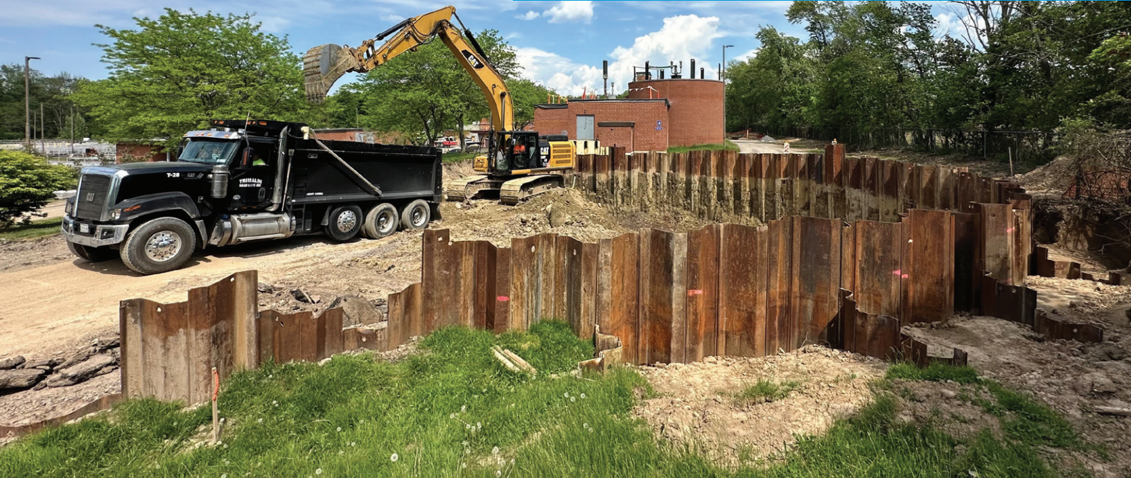
Excavation for the foundation of the new 1.15-million-gallon primary anaerobic digester. The site constraints and soil conditions required the use of sheeting to support the excavation. Photo: Dennis Clough
