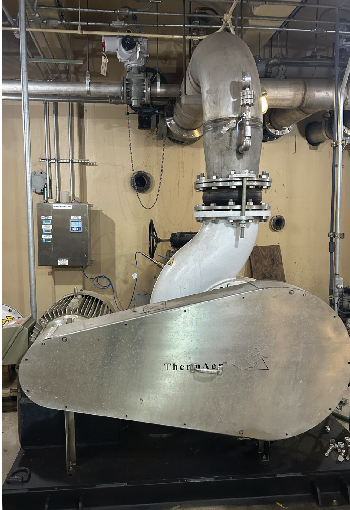
Photo 3. The Thermaer mixing pump typically runs constantly to keep the reactor thoroughly mixed, creating the largest electrical load of the ATAD system. Photo: Tim Carpenter
