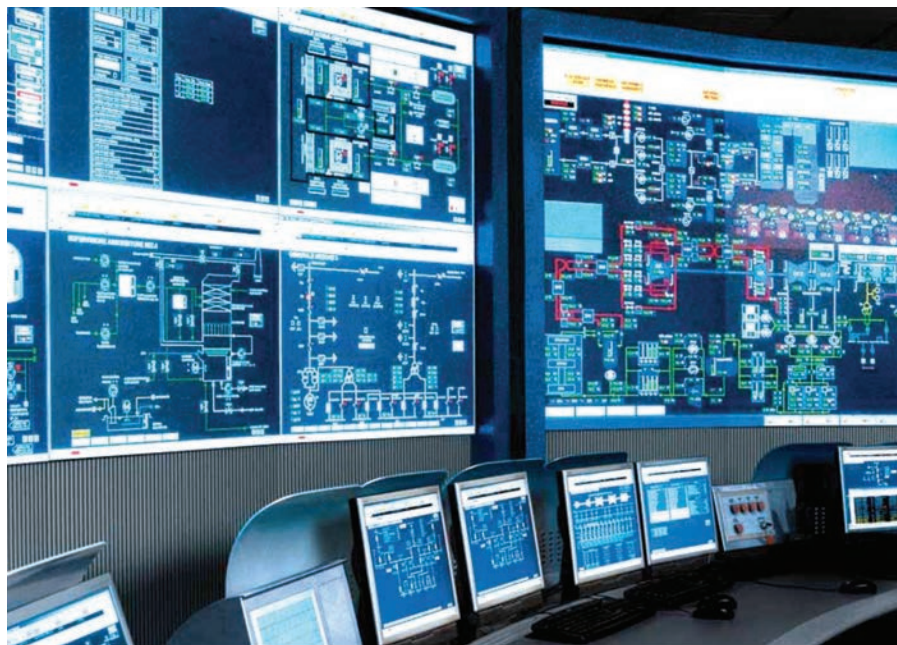
Supervisory Control and Data Acquisition (SCADA) monitors water transport, distribution and treatment. Photo source: Google
