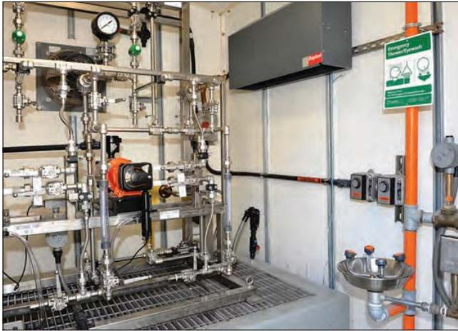
Chemical metering pumps precisely regulate the amount of methanol infused into the denitrification system.
