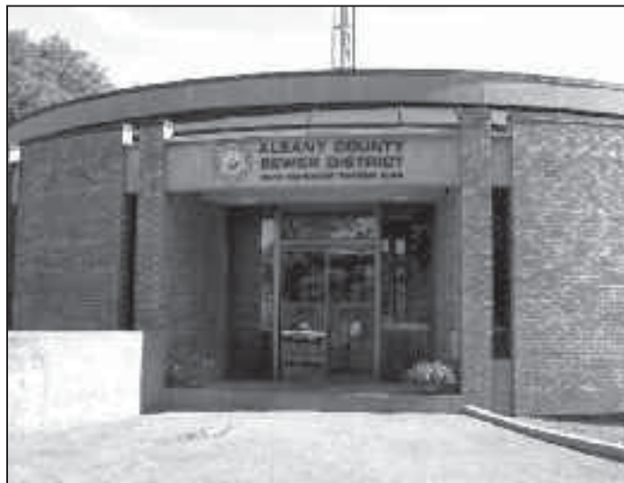
South Plant administration building in Port of Albany, NY
