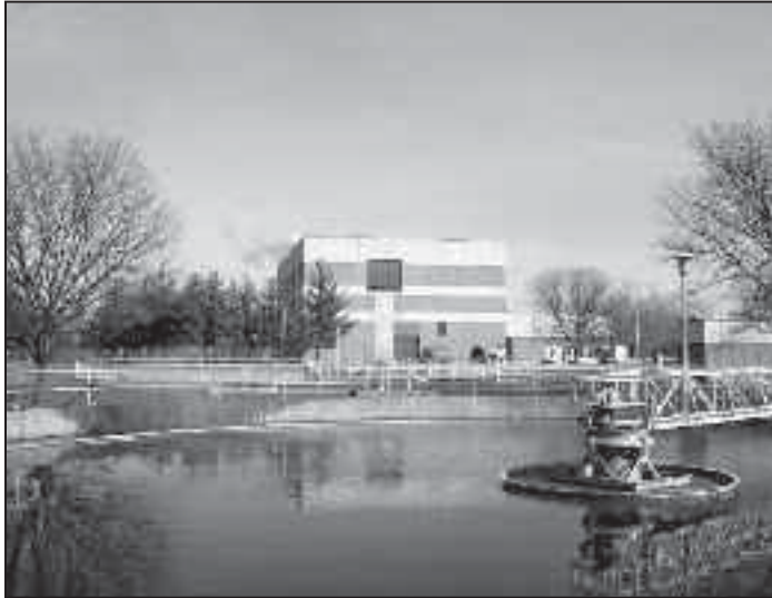
North Plant, Menands, NY
