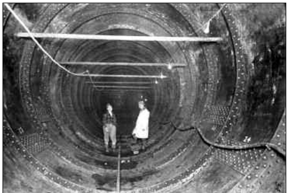
Conditions required the construction of steel lined sections of the Rondout-West Branch Tunnel to prevent groundwater infiltration.
