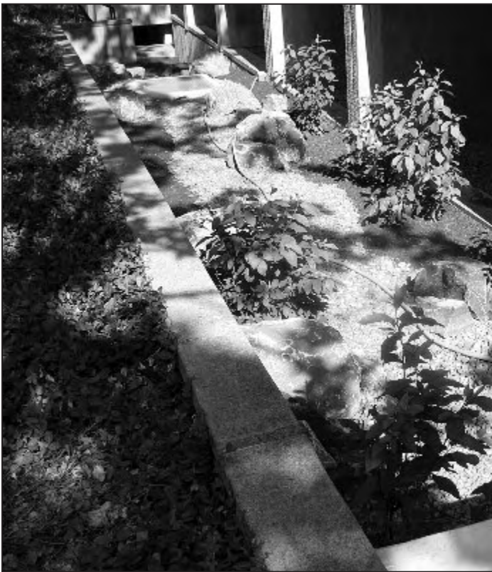
Illick Hall on the SUNY-ESF campus is the location of a new rain garden or bioretention basin made up of soil and plants, where one third of the rainwater from the roof is diverted.
