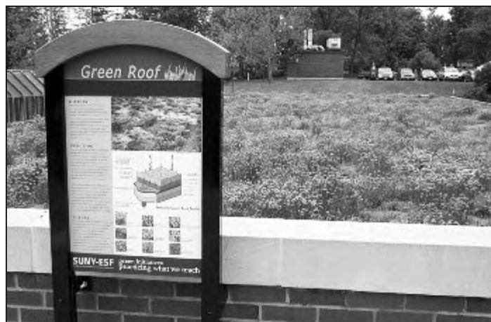
Practicing what is taught: a demonstration green roof design at the SUNY College of Environmental Science and Forestry campus.
