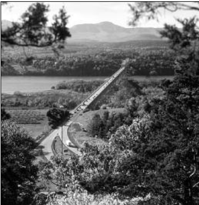
The Rip Van Winkle Bridge, located between Catskill and Hudson, NY, is a cantilever bridge dedicated in 1935 that rises 145 feet above the river to allow passage of freighters to and from Albany.
