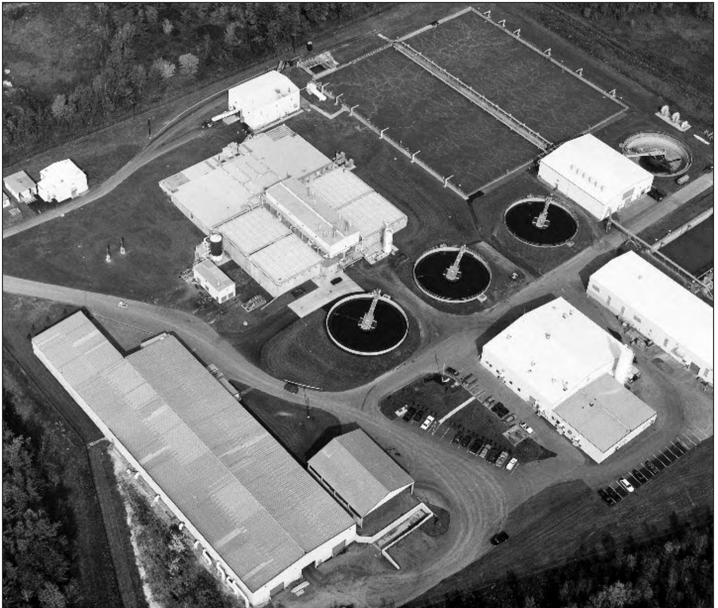
Figure 1. The Anheuser-Busch, Inc. brewery and wastewater treatment plant in Baldwinsville, NY, showing the Bio-Energy Recovery Systems (BERS) facility (center), aeration basins (upper right) and aerobic digesters (far right)
