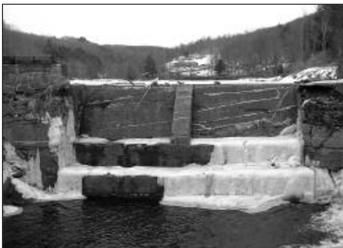
Example of a dam before and after a partial breach project: the remaining low-level drain outlet is discernable along the right edge of each photo.
