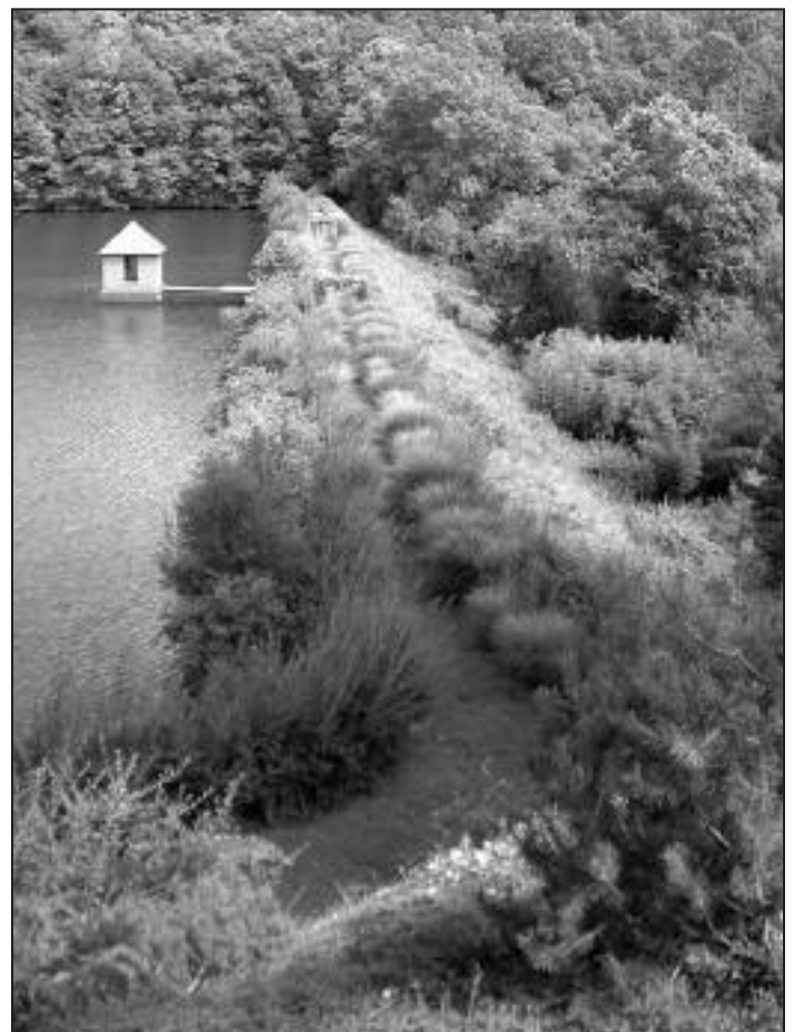
Earthen dams should be maintained with a grass cover.
