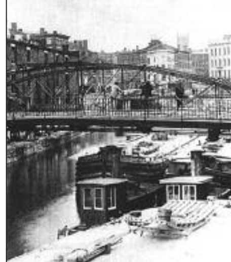
Figure 1. Erie Canal terminus in the past – Commercial Slip
