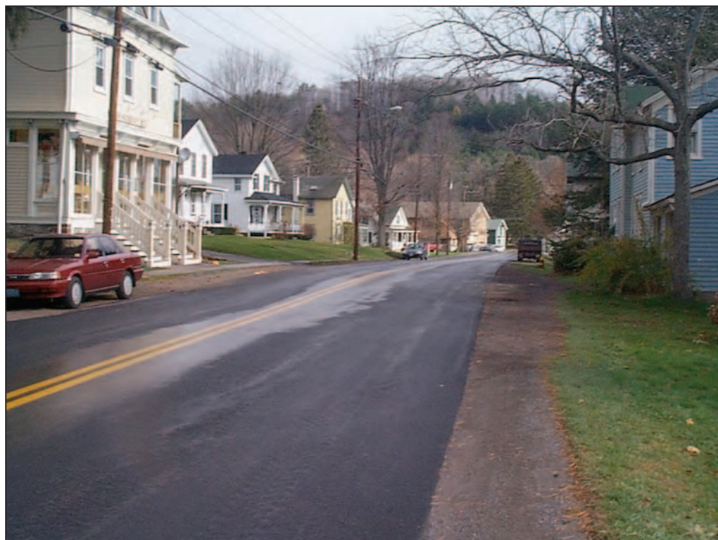
A septic tank/soil absorption treatment system is nearing completion for the Hamlet of Bovina Center in Delaware County.
