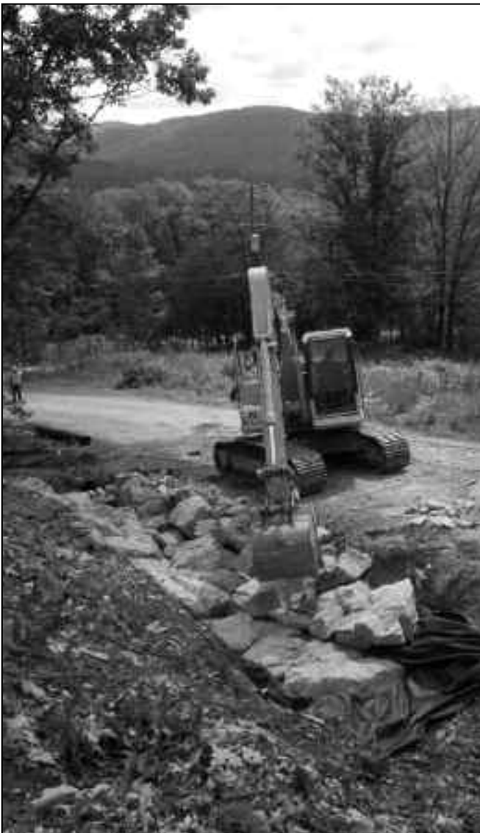
This project to armor ditches, install culverts and plant roadside vegetation to control problematic run off from a steep dirt road onto a state highway and adjoining waterways in the Town of Walton, NY, is one of many Stormwater Retrofit projects funded by the Catskill Watershed Corporation.
