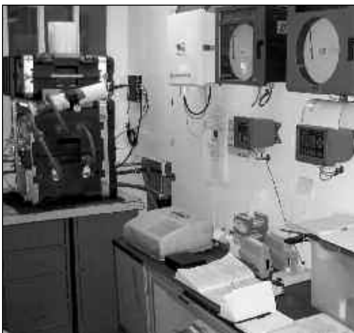
Figure 8: Surveillance at "keypoints," is performed by continuous monitoring equipment found at stations, such as this one, at multiple locations along Catskill and Delaware aqueducts.
