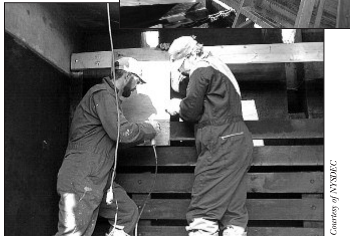
Figures 1a and 1b: Setting up clarifier baffling
