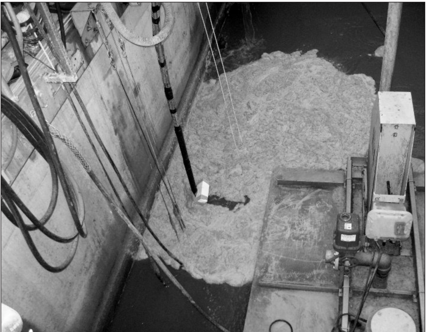
Figure 6: Andes, NY Wastewater Treatment Plant's nocardiofoam removal
