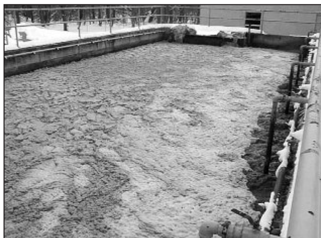
Figure 4: Aeration tank foaming due to nocardioform overgrowth
