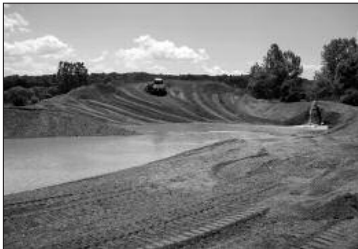
Hydraulically dredged material is being piped into a disposal site on the Champlain Canal. The bulldozer is moving accumulated gravel away from the pipe to make room for more material.
