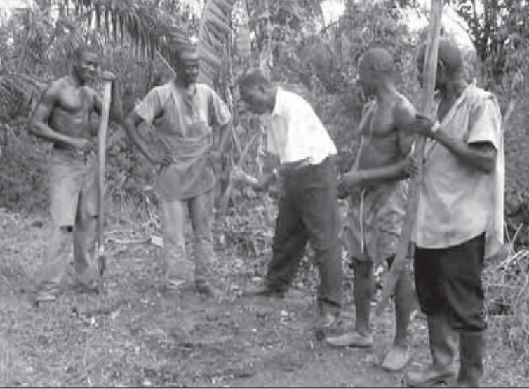
Local Robert Eghan breaks ground for a new well with the laborers and a village elder.
