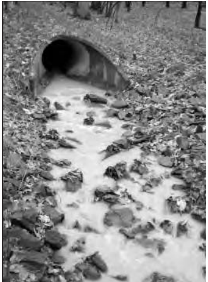
An outlet from a subdivision under construction draining into a flood control basin.
