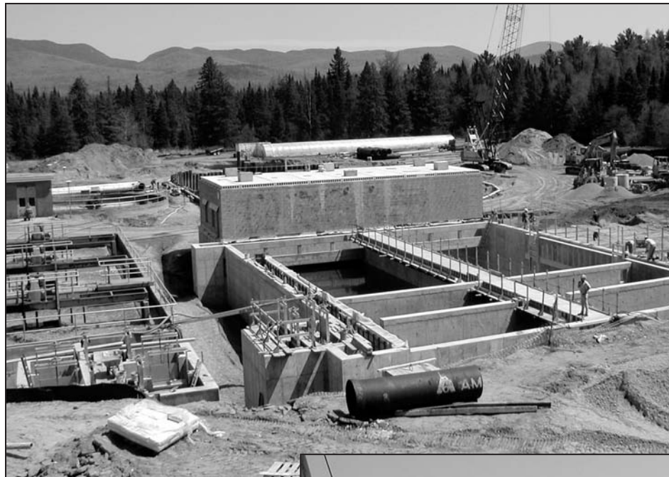
New (80 foot by 14 foot) clarifiers under construction to replace smaller existing ones at Lake Placid WPCP
