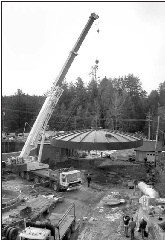
Working on the anaerobic digester at the Lake Placid WPCP
